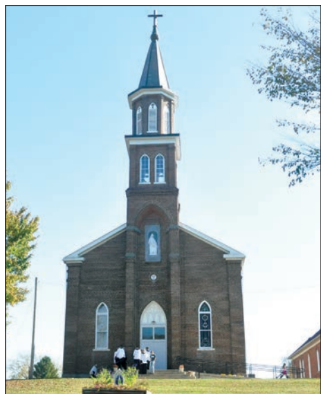
St. Anne Church in Jennings County was built in 1866. As a parish, St. Anne was founded in 1841. Descendants of many of its founding families are still among its members today.
