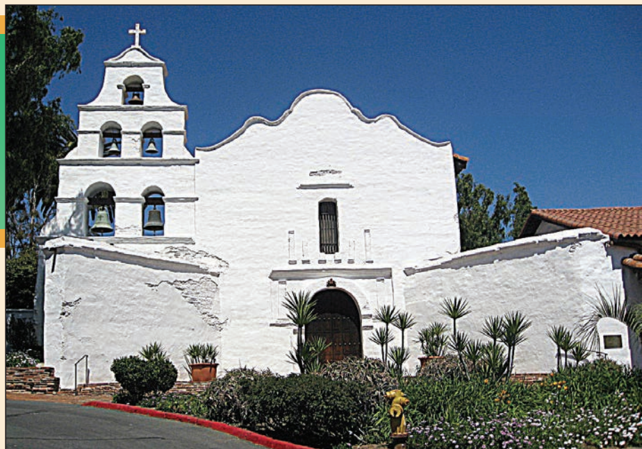
Mission Basilica San Diego de Alcalá, pictured in 2013, was founded on July 16, 1769, and was the first to be established by Blessed Junipero Serra in what is now the state of California. The current church was built in 1931, and is north of San Diego’s downtown area. Blessed Serra, who will be canonized in September by Pope Francis, founded the first nine of California’s 21 missions, most of which remain active parishes. (CNS photo/Mike Nelson)
