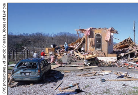
Parishioners salvage items from the debris of St. Luke Church in Salyersville, Ky., on March 3. Six buildings—the church, rectory, an outreach ministry structure, storage building, grotto and picnic shelter—were destroyed by a tornado on March 2. St. Ann Parish in Terre Haute has donated liturgical furnishings and other items to the small faith community in the Diocese of Lexington to help them recover from the destruction caused by the tornado.
