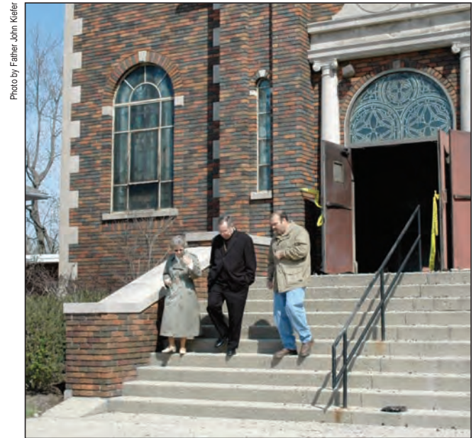
Archbishop Daniel M. Buechlein talks with Franciscan Sister Shirley Gerth, parish life coordinator, and New Castle Detective Mark Stacey after viewing the fire-damaged interior of St. Anne Church on April 10.
