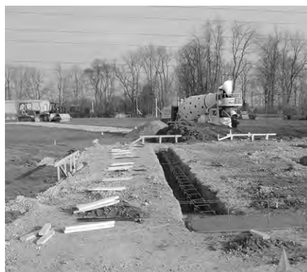
Footings being poured for Prince of Peace Mausoleum
