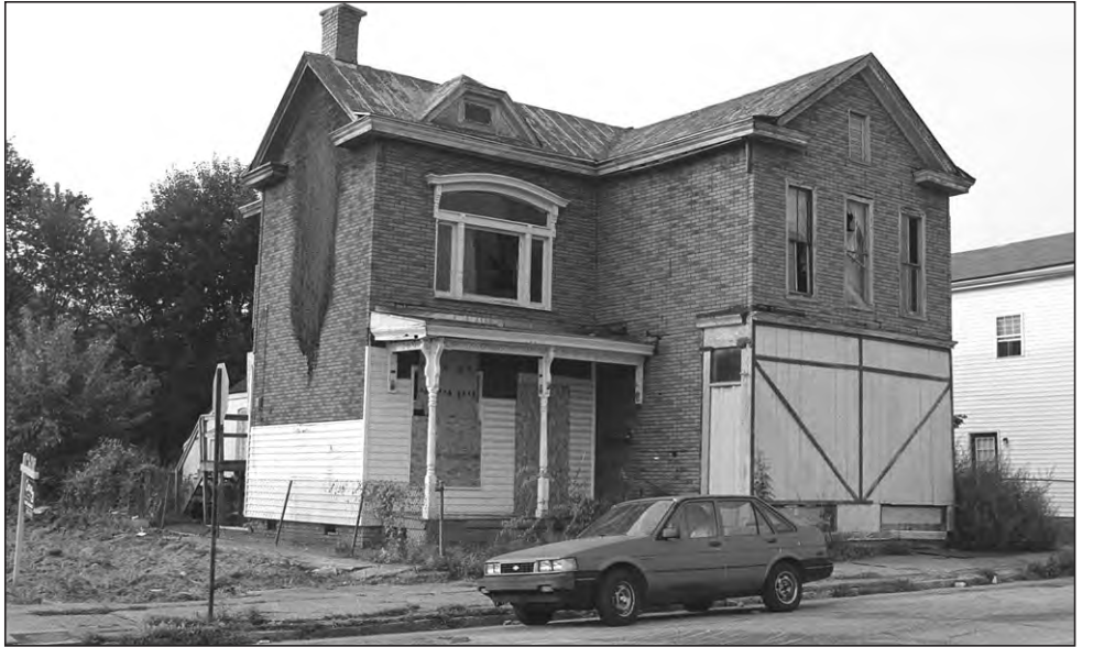
The boyhood home of Joseph Cardinal Ritter, built over a hundred years ago and once a thriving bakery, now sits in severe disrepair. In all likelihood it will be demolished in the coming months to make way for two new houses.
