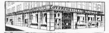
CORNER MARKET AND DELAWARE STREETS Indiana's Oldest Active Savings and Loan Association • In Its 58th Year
